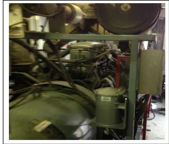
Picture 2 (After Installation-MTU16V2000)
