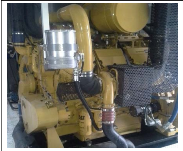
Picture 1 (After Installation-C32) (Actual kit materials not shown)
