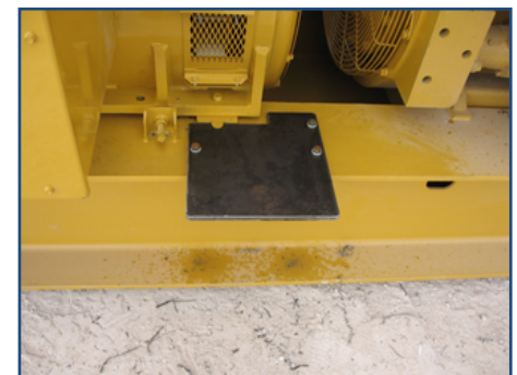
Picture 4: Mounting plate install.- Rail Mounted
